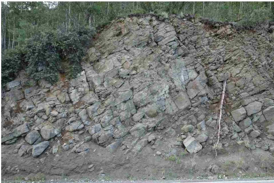
Figure 2.9: Chickaloon formation sandstone in block failure near Milepost 85.5.
